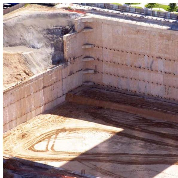
Strut diaphragm walls using metal structures and anchors
