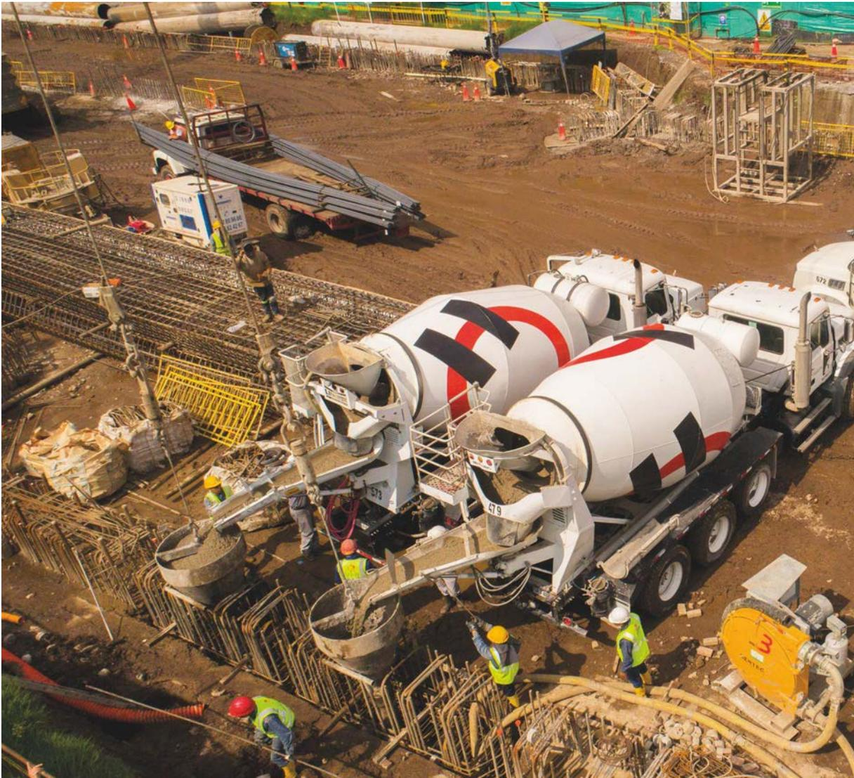
Armed and concrete placement through tremie pipe
