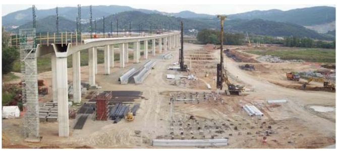
Between February and November 2009, the foundation was made in three piling operations by means of Terra precast piles in structures E-4.1, E-5.1, E-5.3.1, E-7 y E-8.1 of the branch line, Castellbisbal/Mollet, Mollet junction in Castellbisbal (Barcelona).
